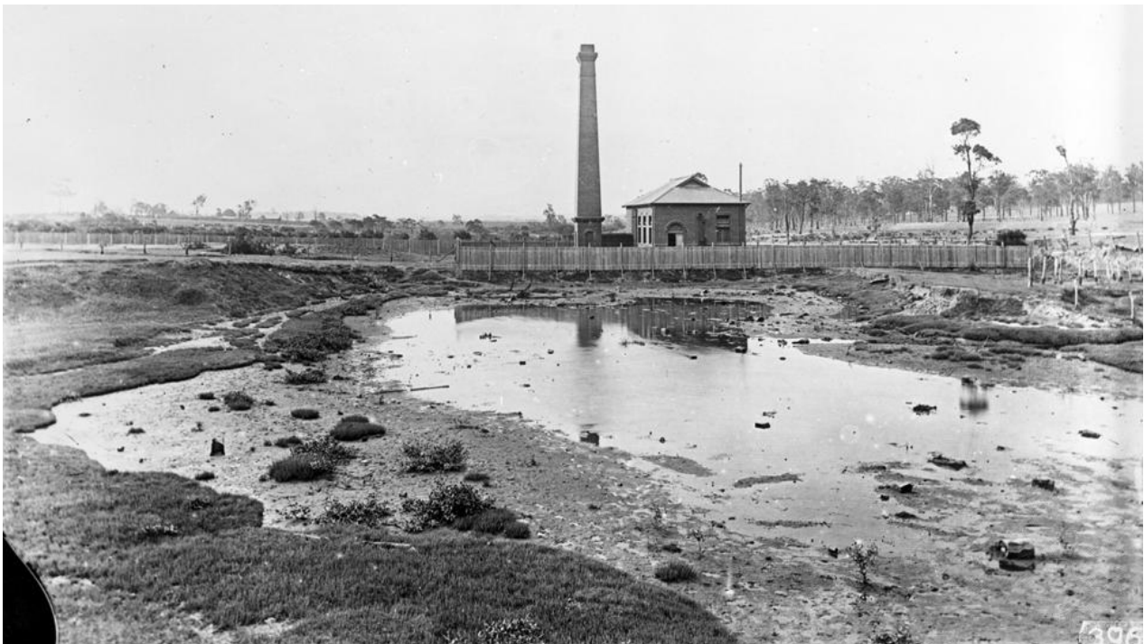
View of the pumping station and vent at the sewage farm in Botany. Unknown photographer, ca. 1900.
