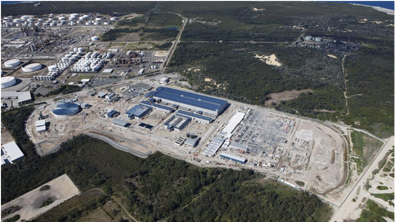
The Sydney desalination plant was constructed between 2007 and 2010. Photograph by Sydney Water, ca. 2009.
