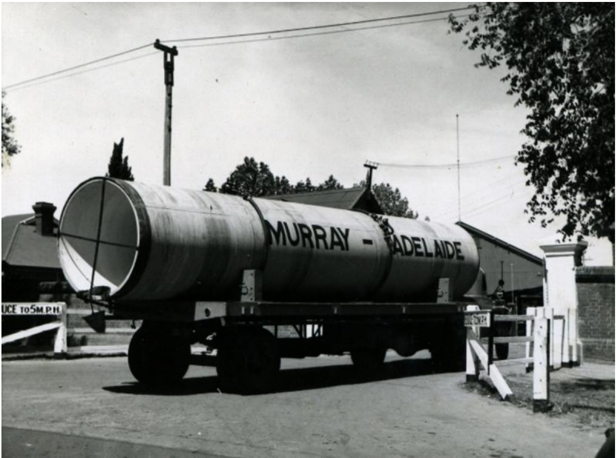
Mild steel concrete-lined pipe leaving E&WS yard in Kent Town as work on Mannum-Adelaide pipeline begins, 1951. Unknown photographer, 1951.
