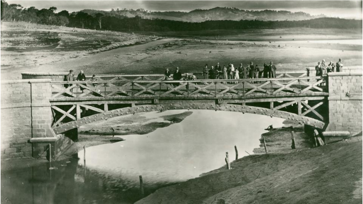
Old Millbrook Bridge, usually underwater, exposed by drought. Unknown photographer, c. 1930–34.
