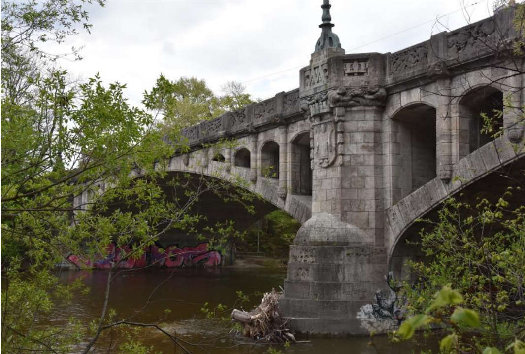
Bridges in Munich, like the Maximiliansbrücke, are constructed with a base made from nagelfluh. Photos © Stefan Bitsch and Alicia Dorner. These works are licensed under a Creative Commons Attribution 4.0 International License.
