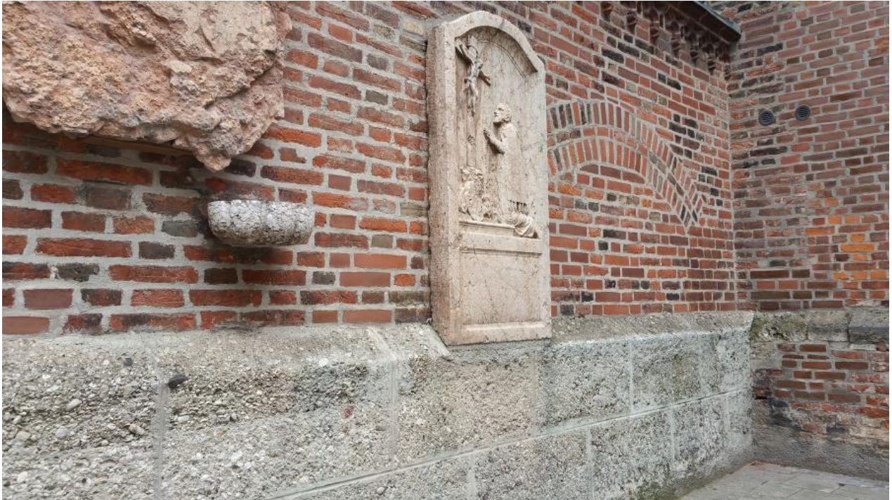
The base of Munich's Frauenkirche consists of nagelfluh and the building façade is made of clay bricks. Photos © Stefan Bitsch and Alicia Dorner. These works are licensed under a Creative Commons Attribution 4.0 International License.
