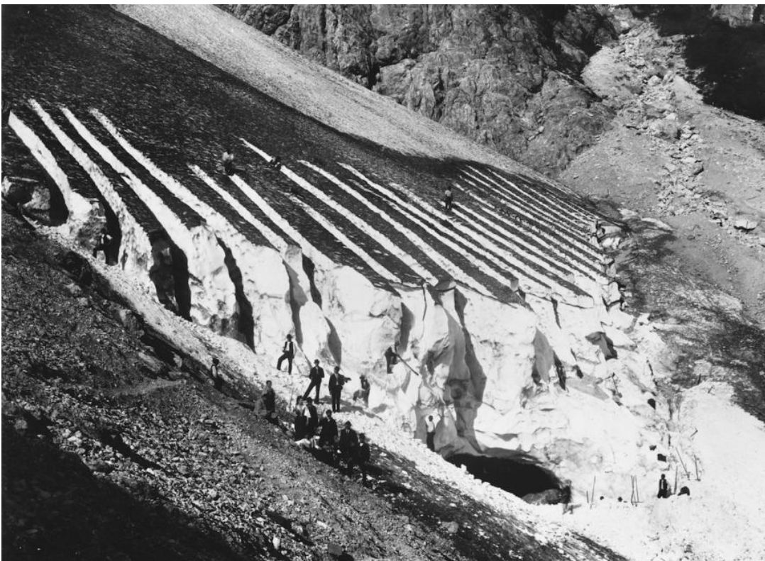
This pictures shows a group working in the ice field at the Birnhorn glacier. Ice blocks were hauled into the valley using wooden chutes. Photo: Deutsches Museum (used by permission of the copyright holder)
