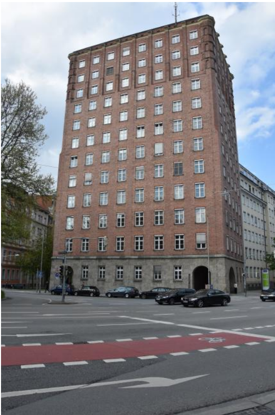
Munich's Städtisches Hochhaus is the city's oldest high-rise building and has a typical composition of a nagelfluh base and clay construction. Photos © Stefan Bitsch and Alicia Dorner. These works are licensed under a Creative Commons Attribution 4.0 International License.
